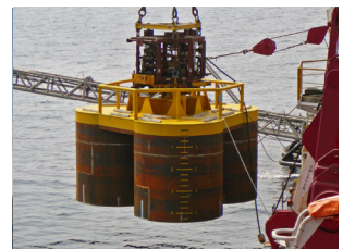
2. Lift and lower SPC to seabed using the integrated suction
