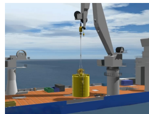
2. Lift and lower suction pile using integrated sp lift frame
