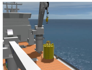
1. Install and lock suction pump on suction pile
