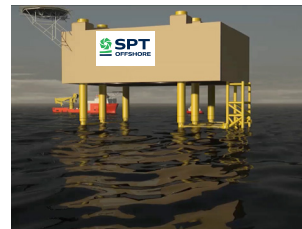
4. Install topsides by floatover or lift
