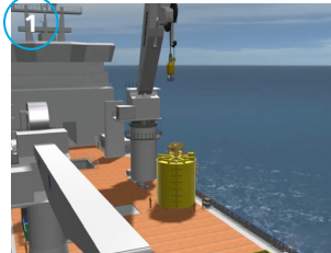
Install and lock suction pump on suction pile
