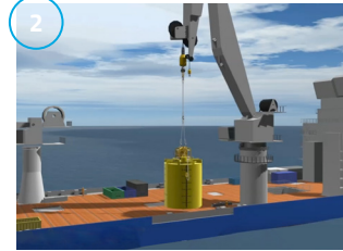
Lift and lower suction pile using integrated suction pump lift frame
