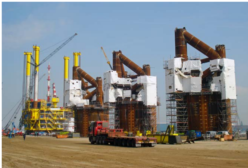
Fabrication of the suction pile foundation for the Centrica F3FA SIP2
