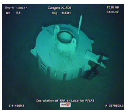
SCR anchor suction pile installed at 1,100m water depth in the Frade field, Brazil
