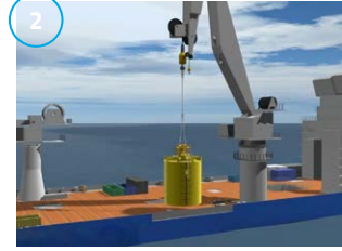
2 Lift and lower suction pile using integrated suction pump lift frame
