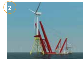
Position and lower to seabed
