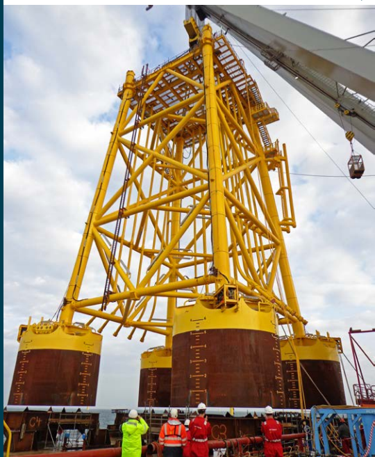
Statoil Dudgeon Substation
