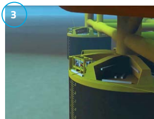
Install suction piles
