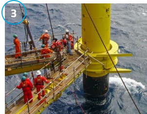
3 Suction operation and welding to bracing
