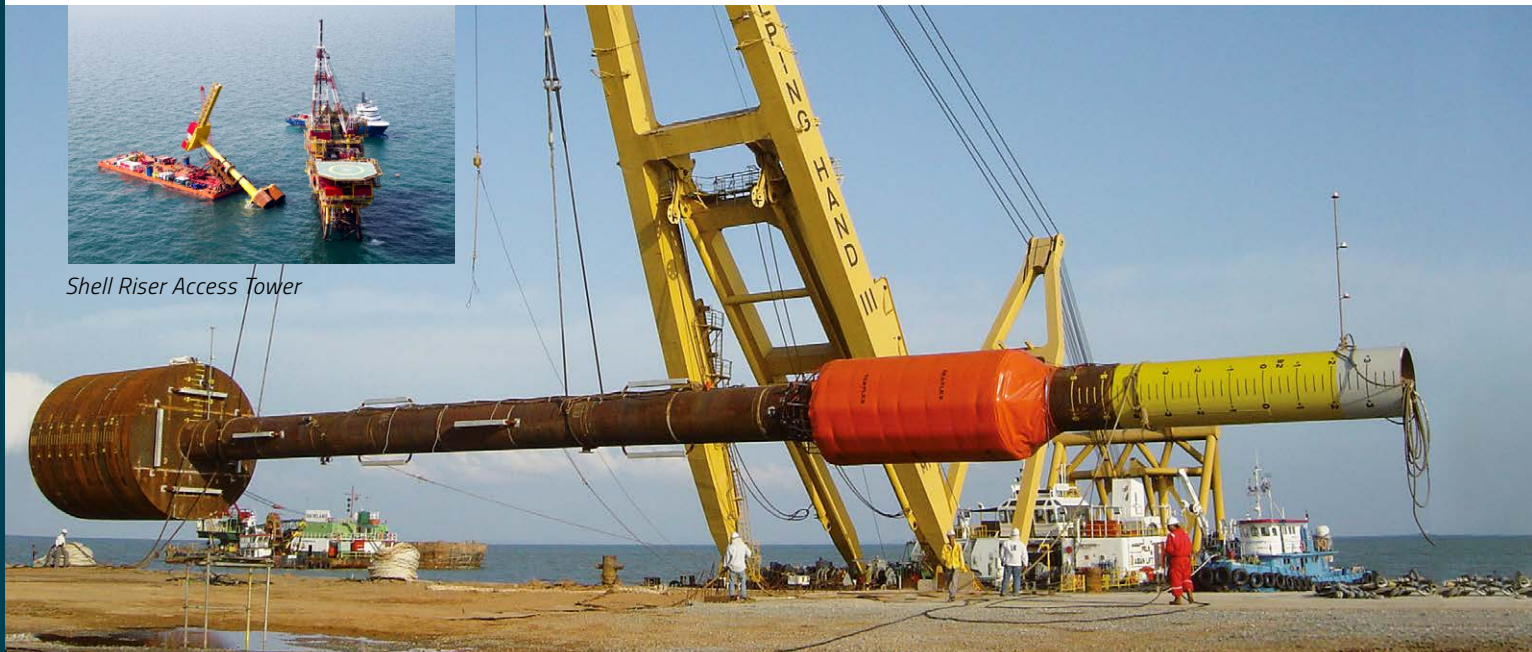
Talisman Bunga Raya Platform Extension
