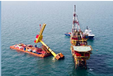
Shell Riser Access Tower
